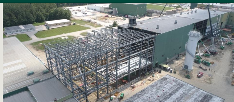
BUILDING EXTENSION - JUNE 2022
